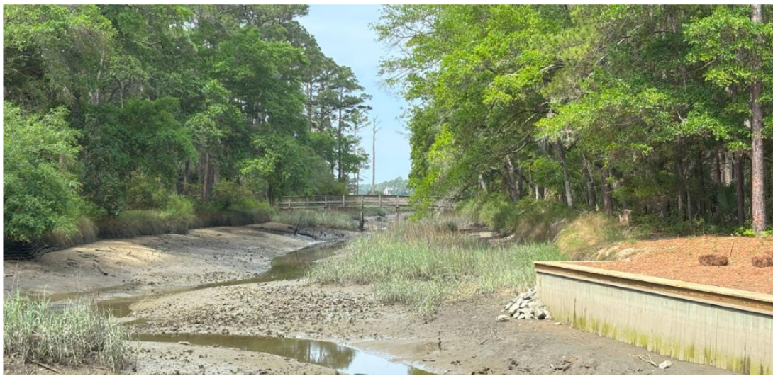
Figure 4. Multi-phase installation of Envirolok on Kiawah Island. Note difference in vegetative cover at different phases.
